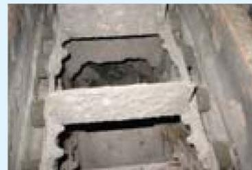
Fly Ash Conveyor: Dust Conveyor Under Boiler
